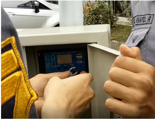
Gambar 6. Pemasangan Solar charge controller portable windsock
