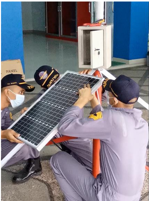
Gambar 7. Pemasangan solar panel portable windsock
