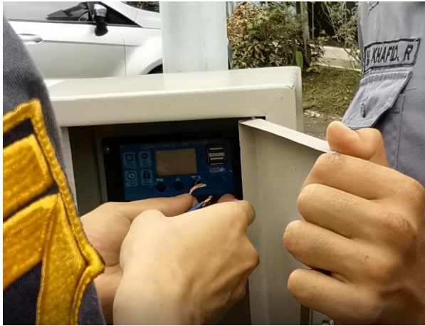
Gambar 6. Pemasangan Solar charge controller portable windsock
