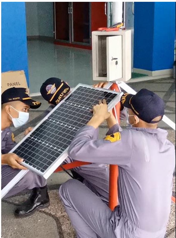
Gambar 7. Pemasangan solar panel portable windsock
