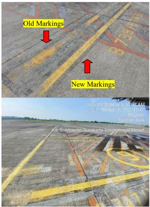
**Figure 3.** Condition of Parking Stand 6 Apron Markings
