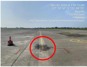
Figure 4. Fluid Spill on Parking Stand 2
