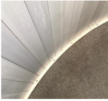
Figure 2. Curtain condition after maintenance
