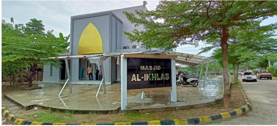
Gambar 1. Tampak Samping Masjid Al-Ikhlâs
